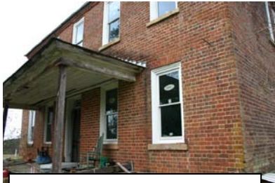
Brick Furman teacherage nearby, now used as a home.
