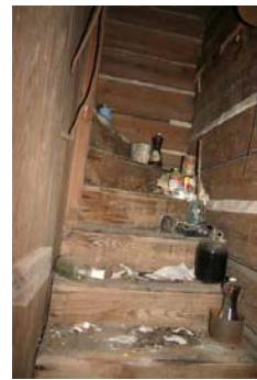
Stairwell in log section
